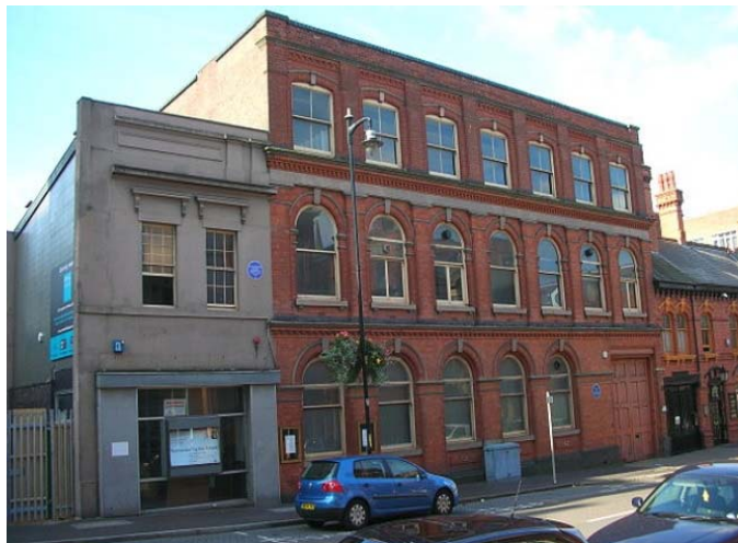
Figure 13 - Original site of the Elkington Plating Works in Birmingham, England, circa 2012.
