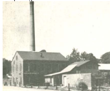
Figure 19 - The former Adams Plating & Mfg. Co. in South Windham, CT circa 1954. 1,4
